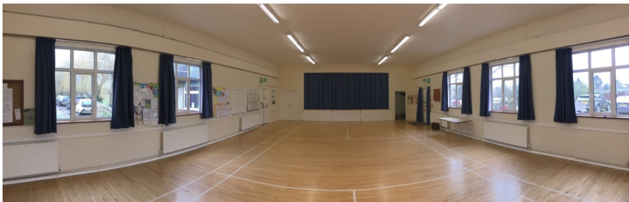
The main hall with recently upgraded LED lighting and party mode uplighting
